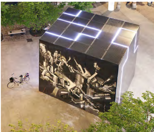
A striking structure creates an iconic entry to the building. The exterior surface of this entry vestibule is comprised of configurable digital walls to mimic the energy consumption, generation, flow, and KPIs of the entire campus in a 3D model , making a strong statement that the Center is not just a building, it is a building with a brain.
